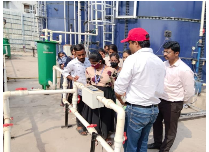
Mr. Sandeep, Engineer at Biogas plant
